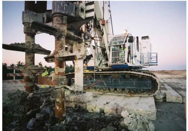
The soils were mixed in situ with predetermined quantities of binder, a blend of Slag and Portland cement. The grout was injected at the bottom of the drilling rods at different rates of pressure and flows to address the peculiar properties of each soil layer.
